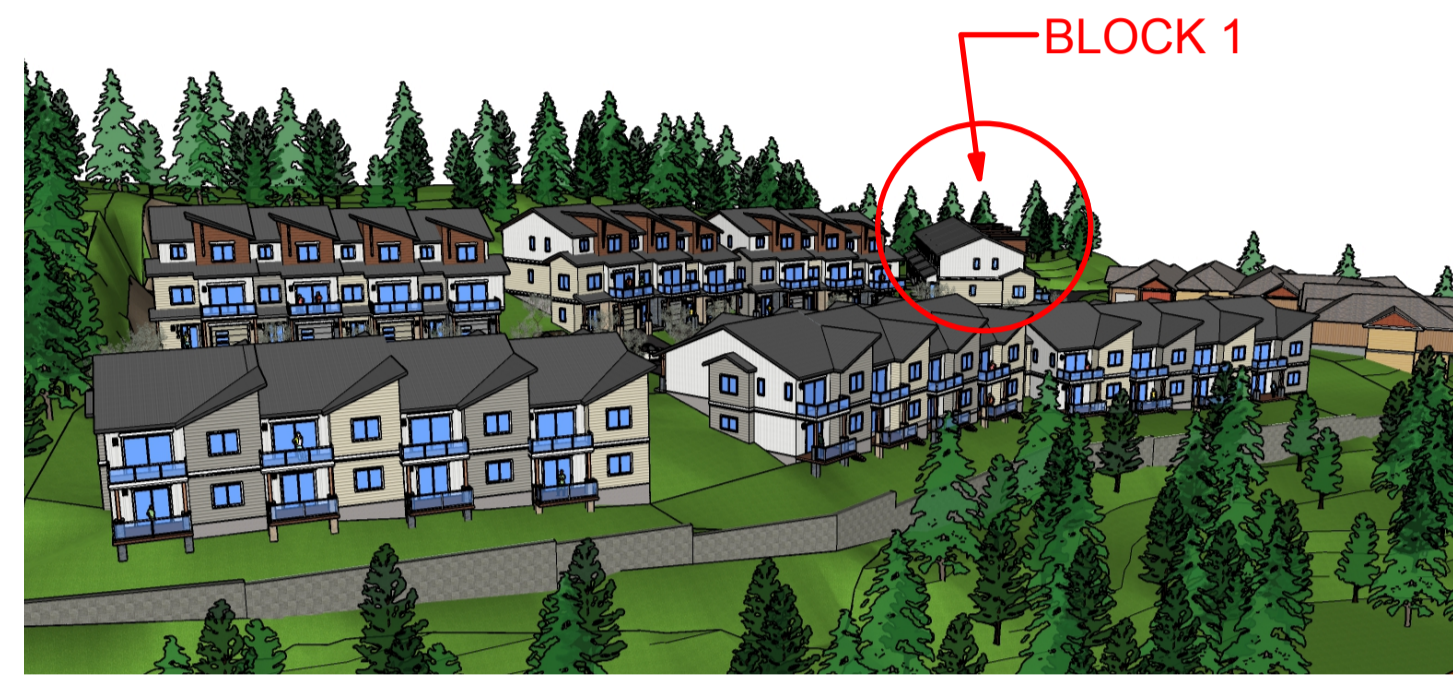
AERIAL VIEW FROM NORTHEAST
