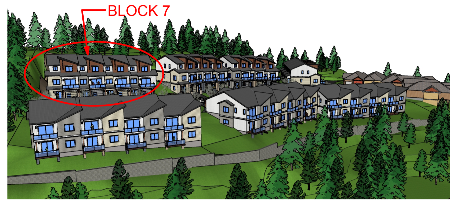
AERIAL VIEW FROM NORTHEAST
